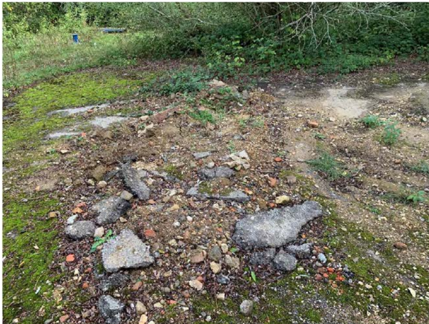
View from within Woodland TPO Area Image clearly shows the ground is asphalt / hard standing.
